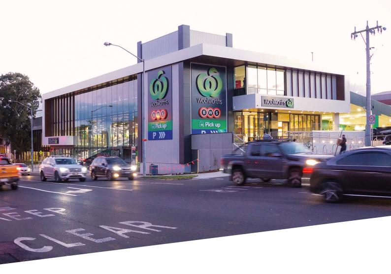
Banksia Street façade however exhibits a slightly different IGU makeup, intentionally making the south facing facade opaque in appearance, these IGU's combine the use of 6mm Toughened ColorSmart™ Black panels, 12mm Argon Gas filled IGU Space and 6mm Toughened EnviroClear®.
